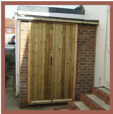
The newly completed lean-to
