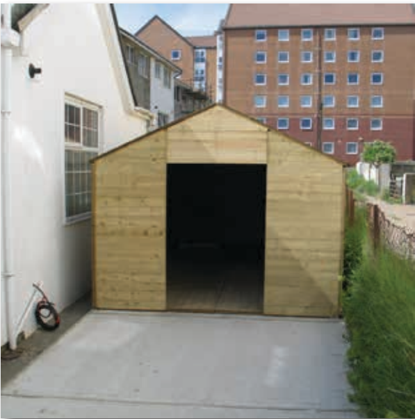
Progress on the workshop so far
