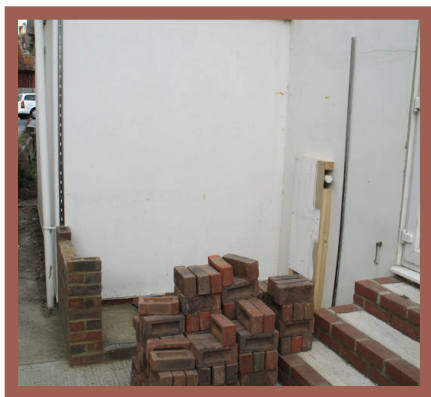
The first few rows of the new lean-to
