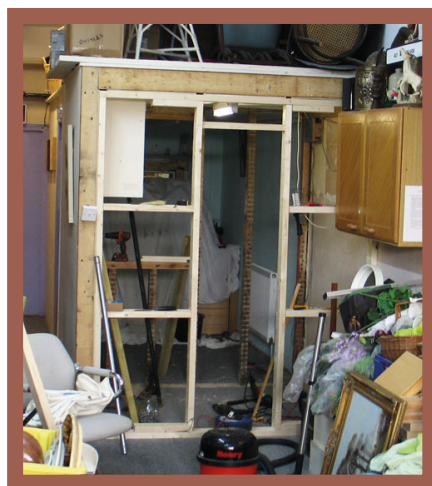
The studwork for the extended dressing room
